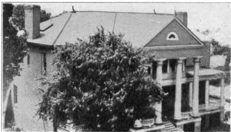
Old Marine Hospital at Norfolk, Va., the first Marine Hospital owned by the Marine Hospital Service, purchased from the State of Virginia in 1801.
